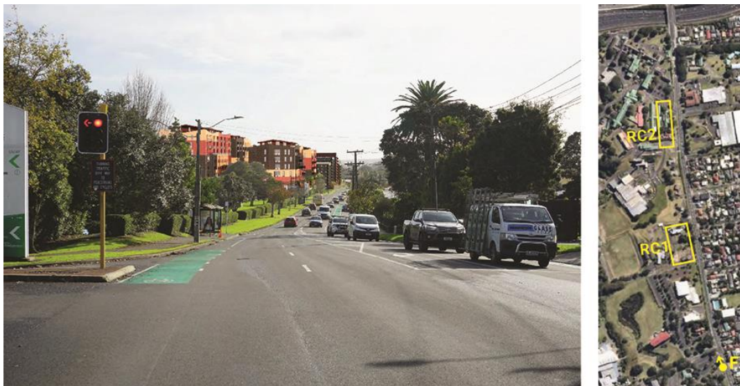
Figure 2: Looking south along Carrington Road from the intersection with Sutherland Road to the RC2 development in the foreground and the RC2 development in the background. Image source: Maungārongo RC1 and RC2 Assessment of Landscape Effects.
