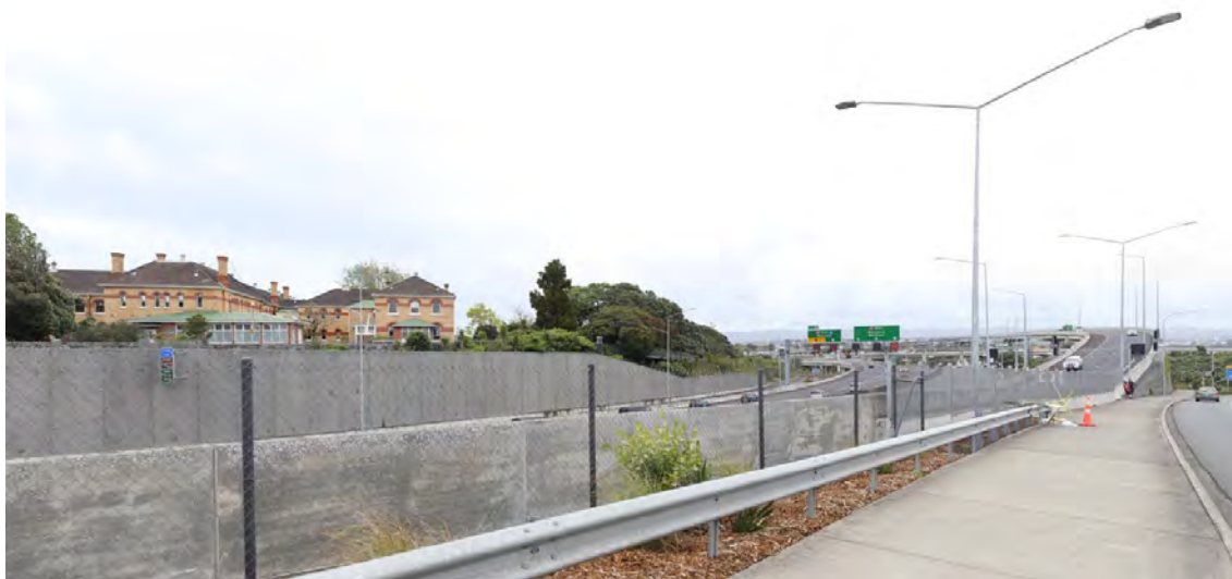
Figure 2: Photograph showing the context of the site to the North-Western motorway and Waterview elevated overpass structures.
