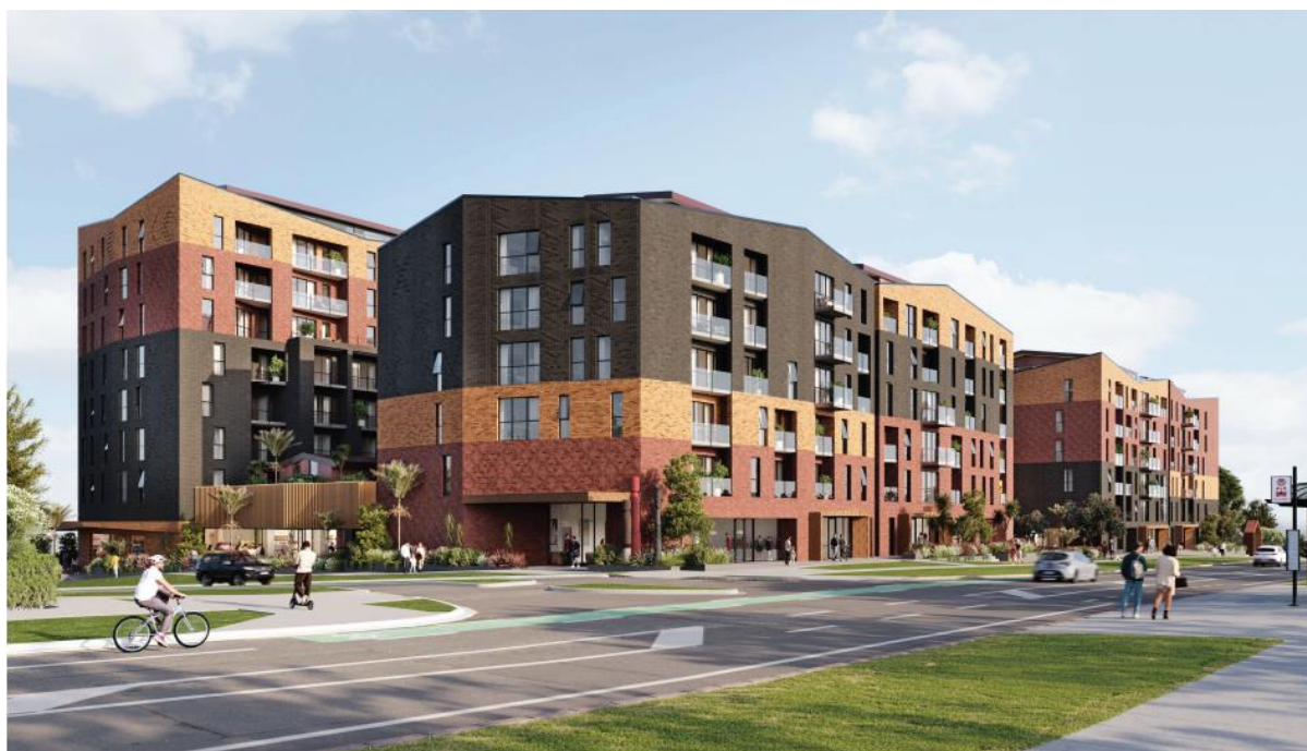
Figure 2: Render of the Maungārongo RC1 buildings as seen from Carrington Road. Building 1 East is in the foreground with the western tower of Building 1 behind. Building 2 is to the right of the picture. Image source: Maungārongo RC1 Urban Design Statement.
